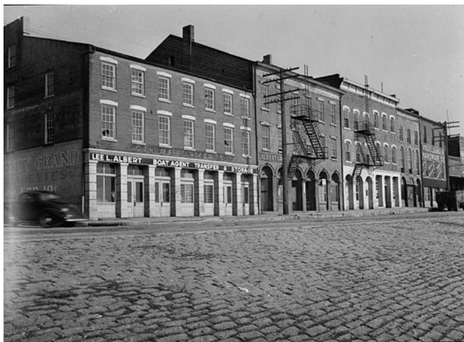
“Row of Early Buildings Facing the Wharf” on Water Street between Themis and Broadway, Cape Girardeau, 1936. Historic American Buildings Survey, Library of Congress Prints and Photographs Division
