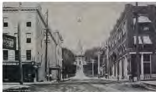
Main and Themis, downtown Cape Girardeau, looking west—early 1900s
